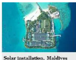
Solar installation, Maldives
